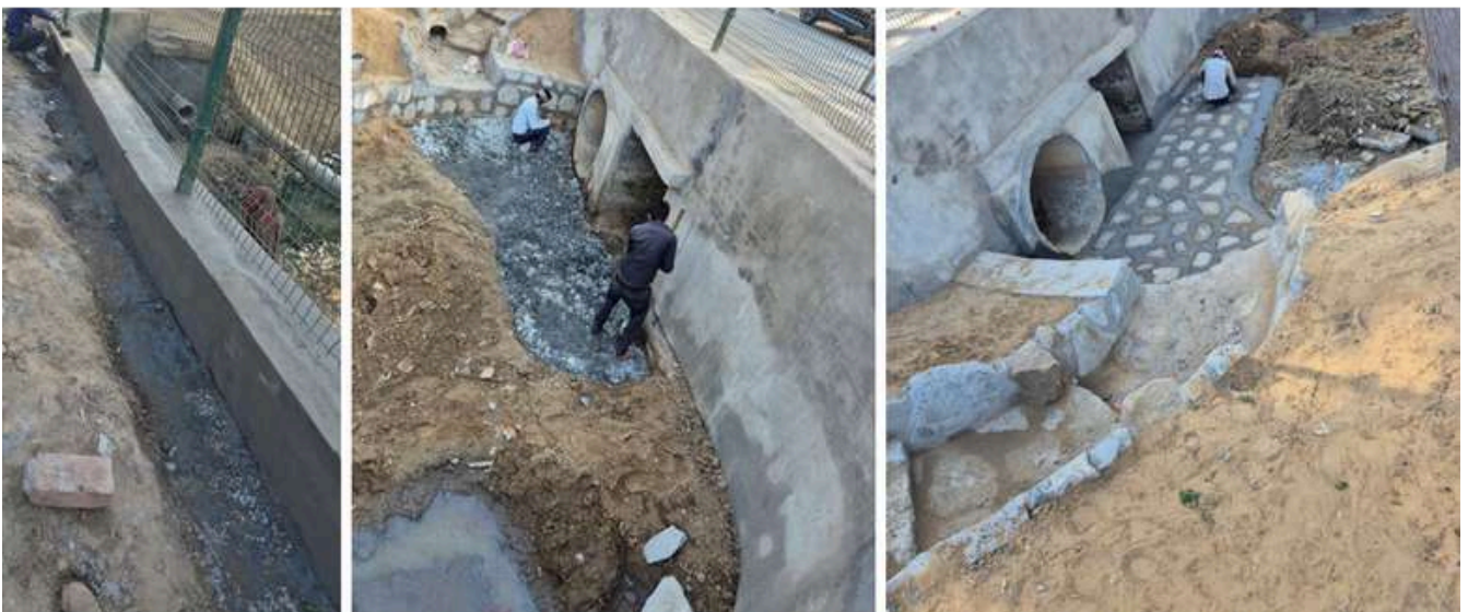
Apron construction at the drain outlet to prevent erosion at the outfall area
