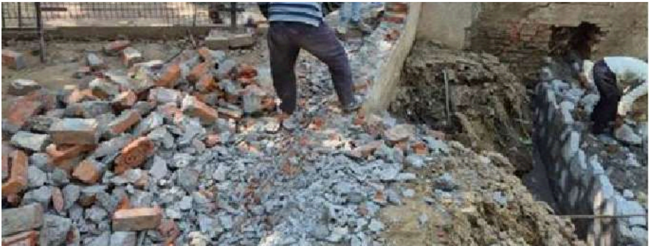
Breaking the wall and building culvert with the malba waste.
