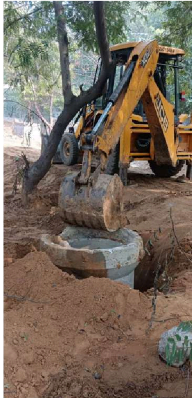
Digging a recharge Pit & Insert a pipe
