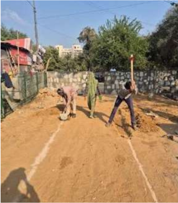
Breaking the wall and building culvert with the malba waste.
