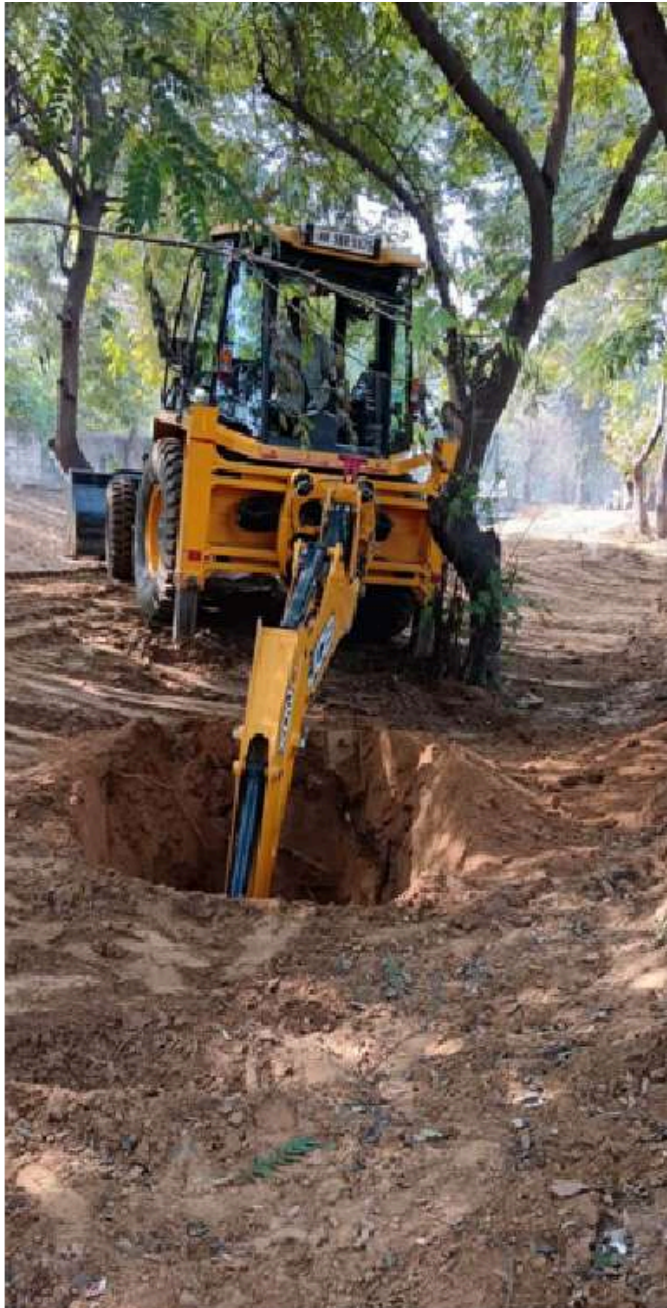
Digging a recharge Pit & Insert a pipe
